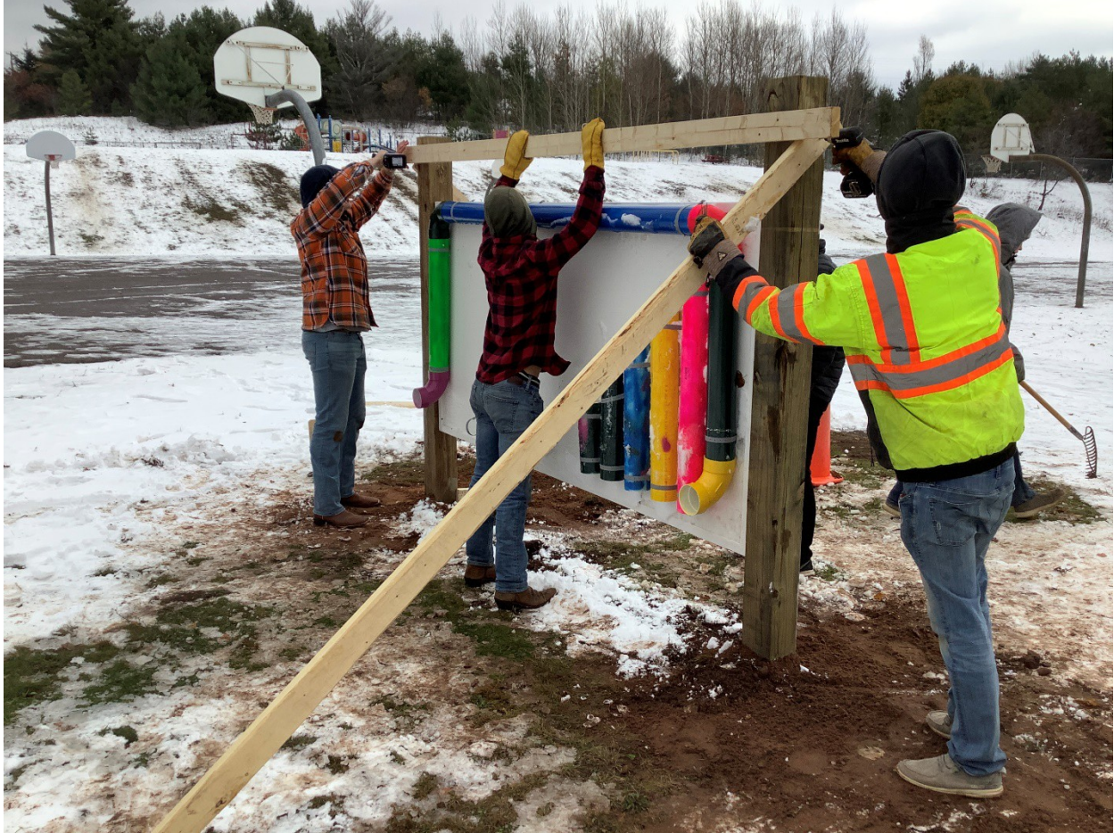
Copper Country ISD Career & Technical Education students remove supports after setting the posts for the new CORE Board created by CTE students and available on the Barkell Elementary playground that will be used by students to assist and promote communication.
